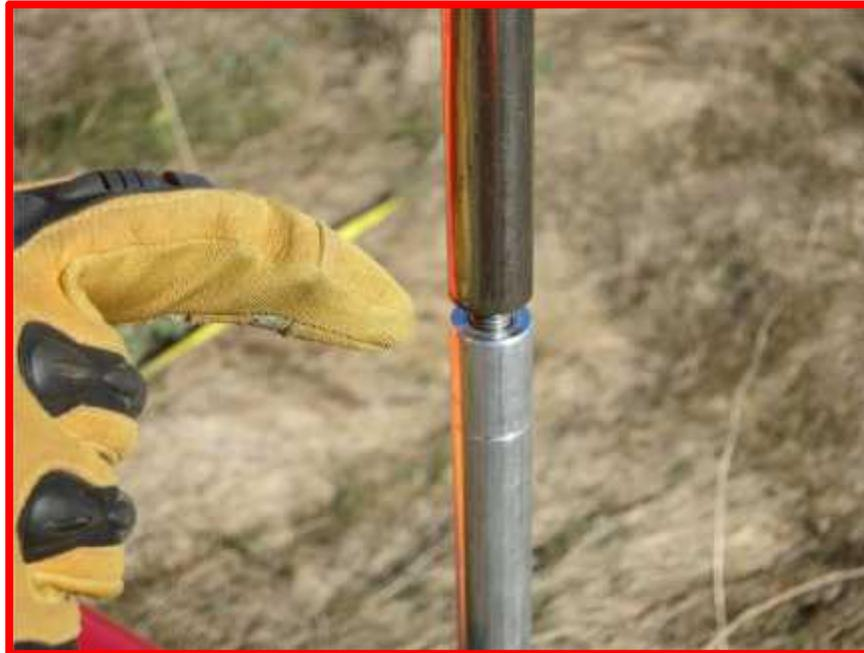
**Figure 12.** Do not allow the monument assembly sections to become separated while striking
