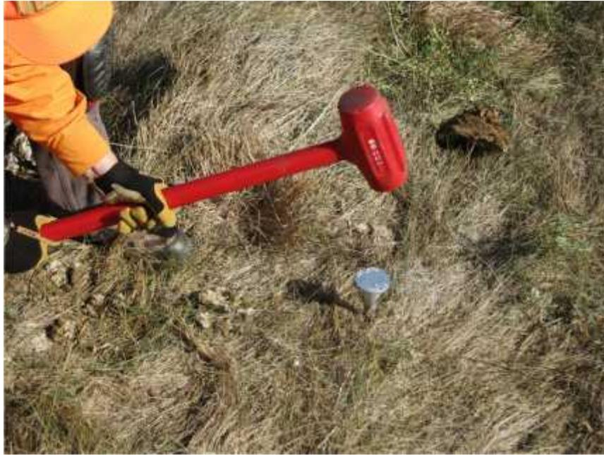
**Figure 14.** Use a sledgehammer to seat the cap and drive the rod to the desired position
