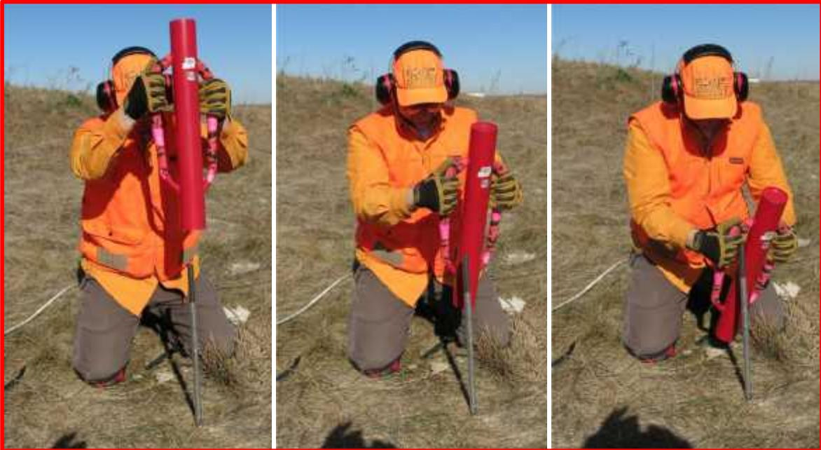
**Figure 13.** Do not lift the post driver above the top of the rod during the striking motion as the worker could injure their leg or hand
